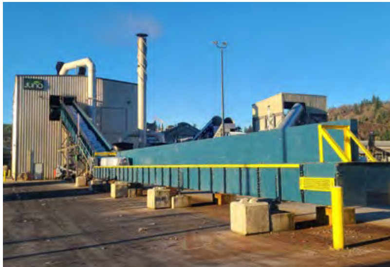
An existing mixed waste processing facility in Oregon
