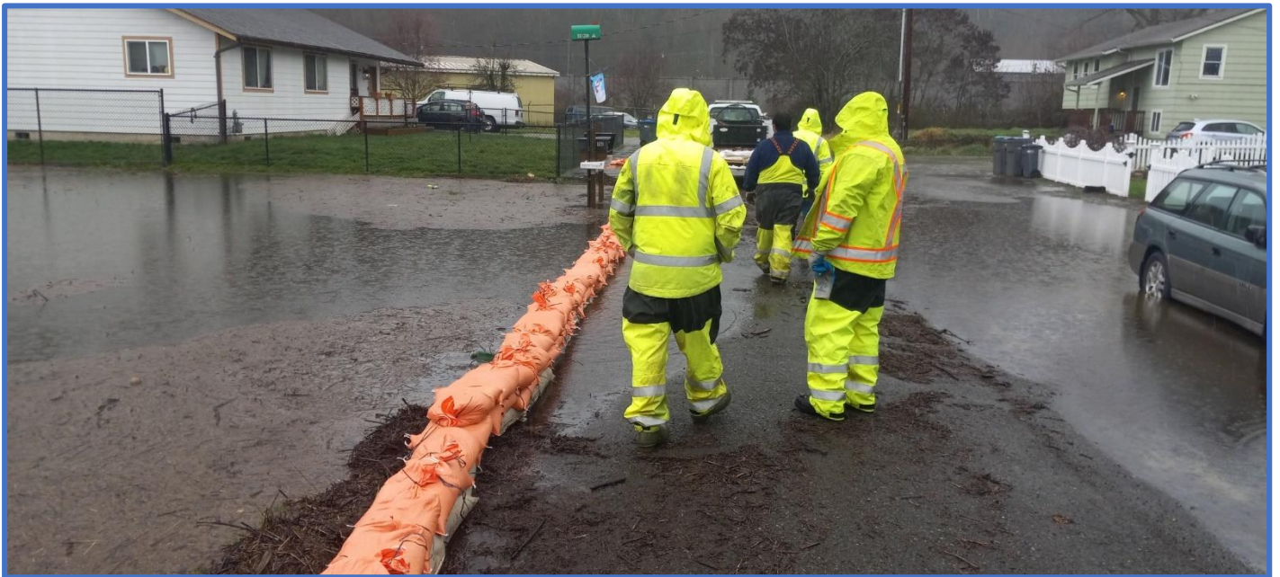
City Public Works staff typically sandbag vulnerable neighborhoods in northern Algona to reduce the impacts of seasonal flooding. Sandbagging is not a permanent solution. Significant infrastructural improvements are necessary to maintain homes and businesses.
