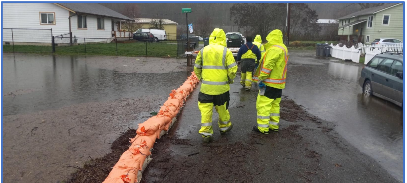
City Public Works staff typically sandbag vulnerable neighborhoods in northern Algona to reduce the impacts of seasonal flooding. While sandbagging is not a permanent solution, significant infrastructural improvements are necessary to maintain homes and businesses into the future.
