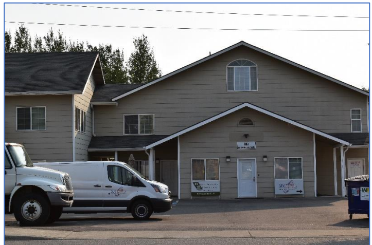
The Mixed-Use Commercial zone is a walkable area with a mix of low-density homes and businesses. Some businesses in the C1 zone have the appearance of a residential unit like Southgate Electric and SeaTemp on Washington Boulevard.
